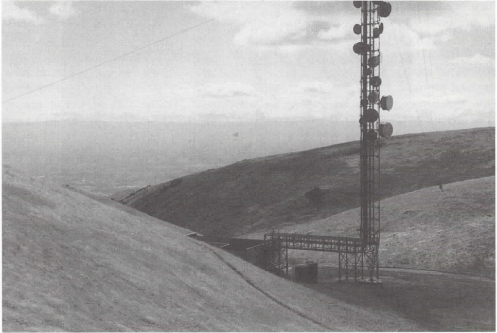
Figure 1.13 Bridge carrying RF power (through a transmission line; see Chap. 13) from the transmitter building to the base of the tower, and then up the tower.
