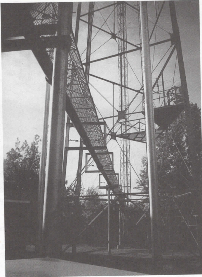
Figure 1.14 RF transmission line, which appears to the layperson as water pipes, carries the RF energy from the UHF transmitter up to the antenna on top of the tower.
