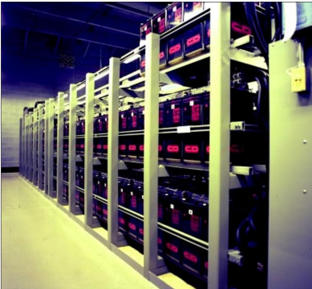
Large battery banks can serve as effective backup or can be used to assume some of the grid load during peak usage periods, a practice called *peak shaving*. Photo courtesy Caterpillar Inc.
