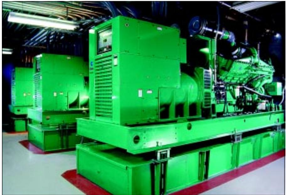
**A generator should be sized to 60 percent of actual load, as loads will tend to increase over its lifetime. Proper loading will also increase its lifespan, ensuring a good return on investment.**
